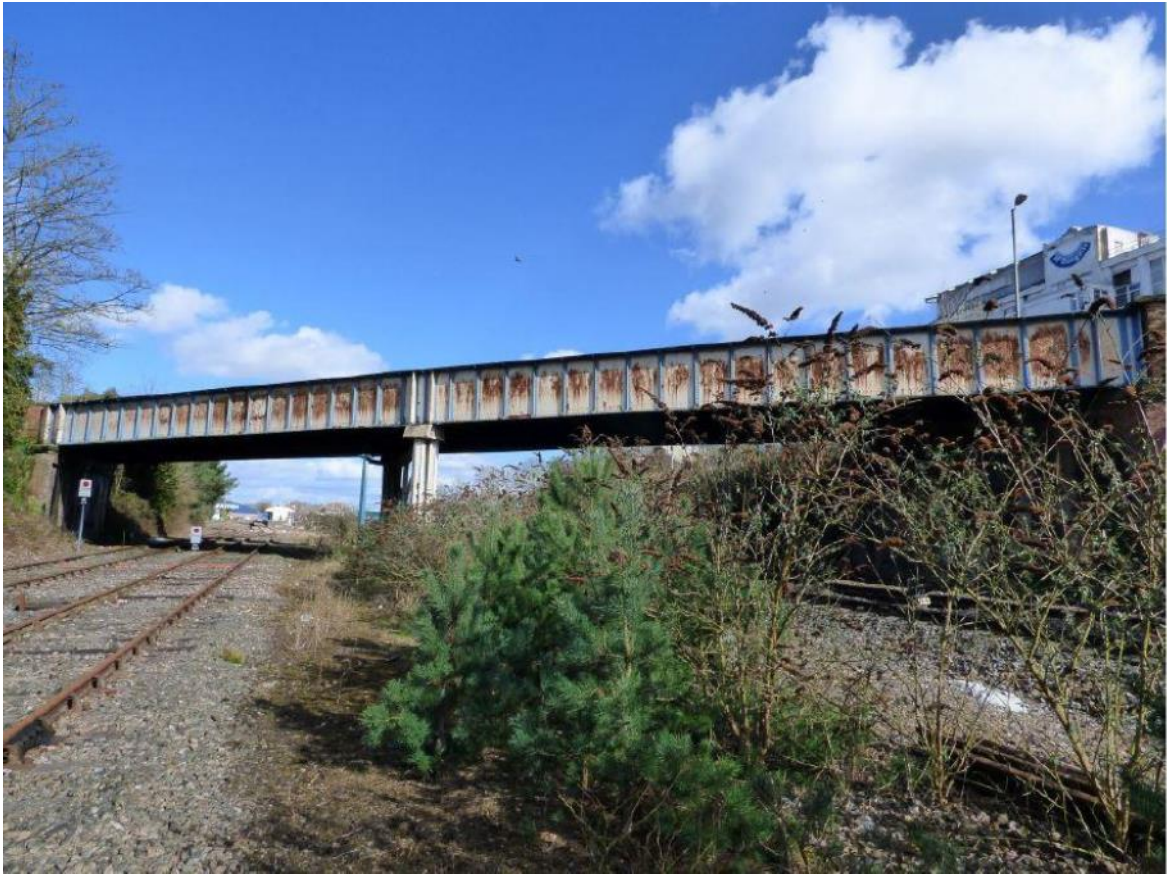
West elevation from track level.
