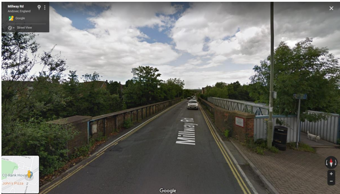
View looking North over Millway Bridge.
